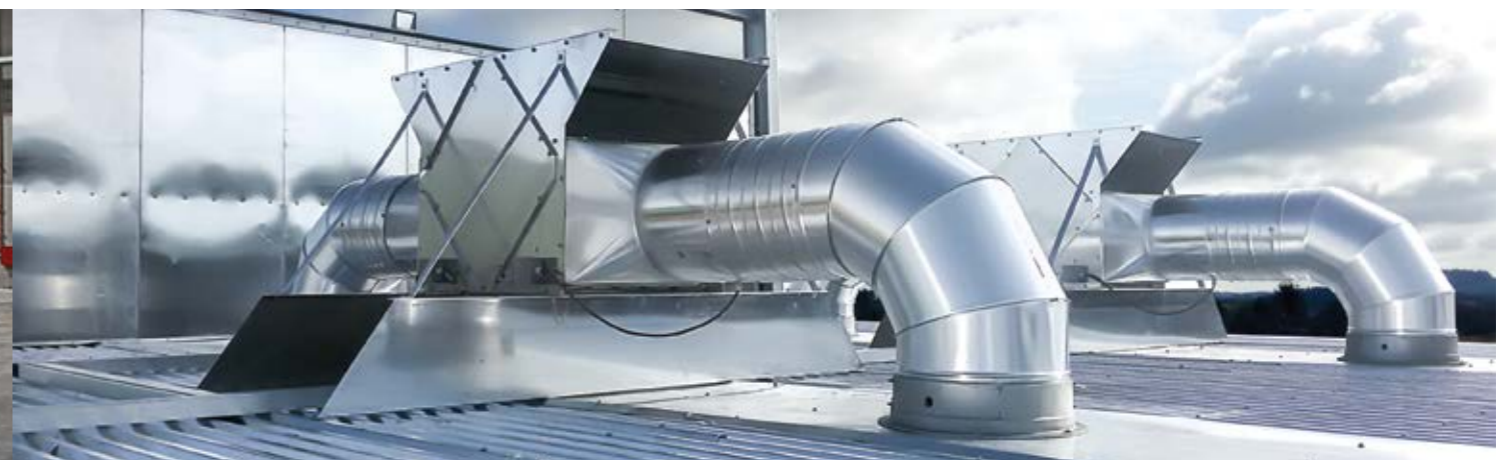
Pictured: Cross-flow heat exchanger
